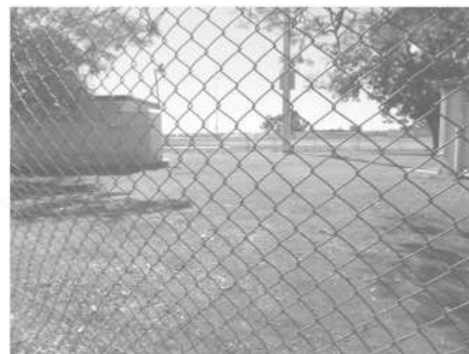
NEW FENCING AROUND THE SITE
